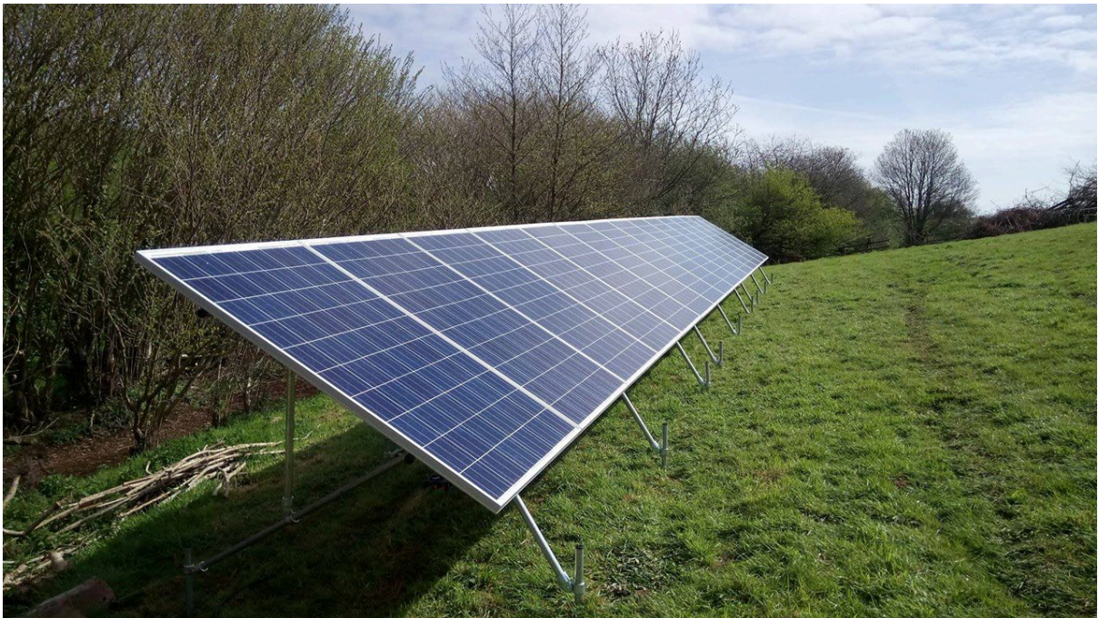
Typical structure layout using ground poles
